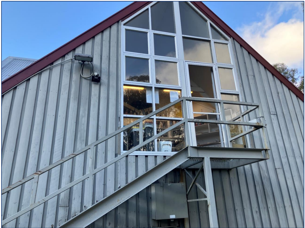
Figure 6 | Non-compliant external balustrade from second floor staff accommodation common room (Source: Department's Site Inspection 2023)
