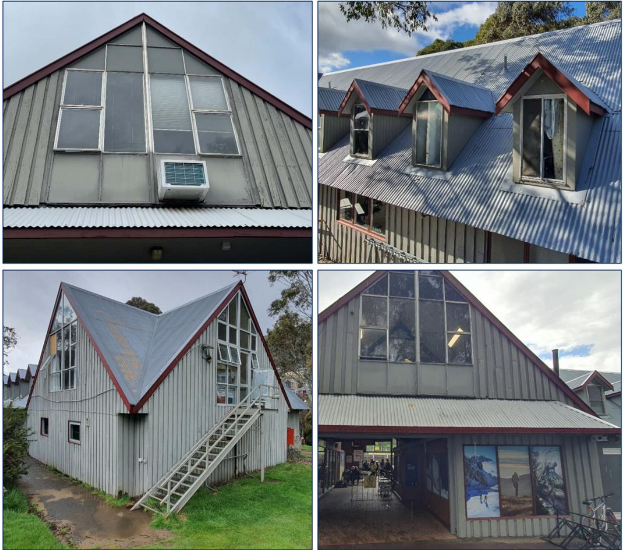
Figure 3 | Areas of the VT that require roof sheeting and window replacement (Source: Applicant's SEE)
