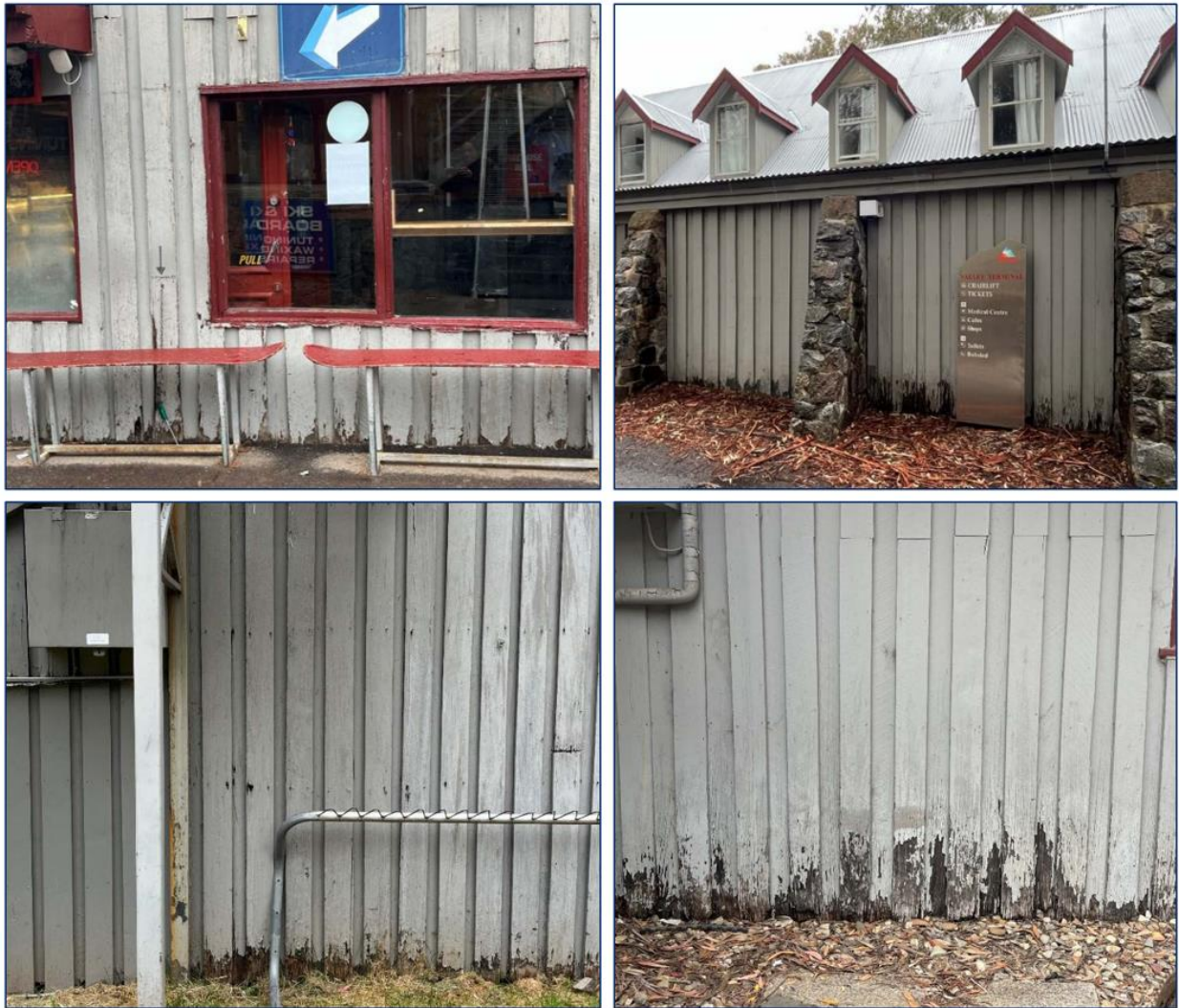
Figure 2 | Areas of VT that require timber cladding replacement due to rotting and deterioration (Source: Applicant's Statement of Environmental Effects [SEE])
